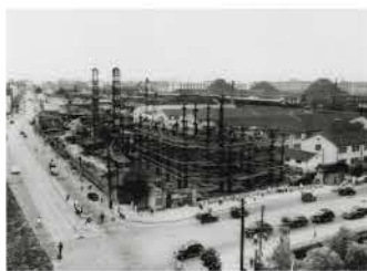
1949 第一鉄鋼ビル起工 Dai-Ichi Tekko Building under construction
