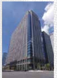
Current TEKKO BUILDING.
