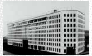
TEKKO BUILDING (No. 1) soon after completion.
